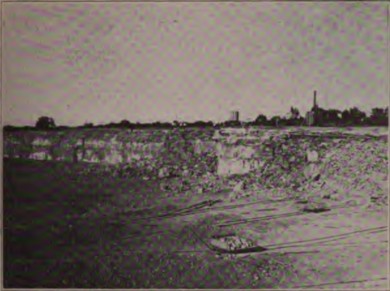
Limestone Quarry, Tiffin, Eastland County
